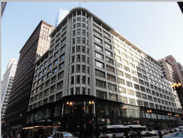
Louis Sullivan. Carson Pirie Scott & Co. Building. 1899 -1903
