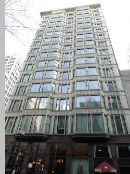
Burham & Root. Reliance Building (Brunham Hotel) 1891-1895
