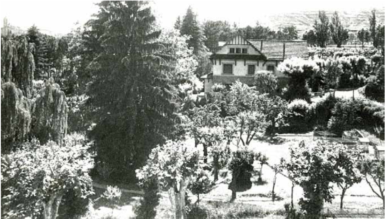
■ The owners' tower, and the garden that circled it, at the Can Riva factory (Les Masies de Voltregà). The Oliveras de la Riva family, in charge of the factory for many years, spent long periods of time there. The current state of the gardens is not the same.
