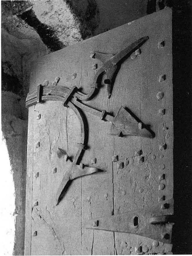
Entrance door. Details of the treatment based on agricultural utensils and pieces of wood joined on boards.
