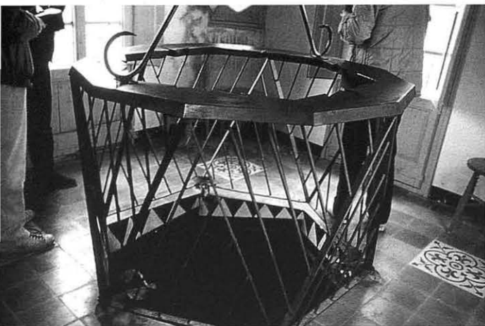
Interior of the building. Details of the bannister and the stair-well. A plank out in the form of a saw, held up by light metallic elements, forms the circular balcony that looks over the well.
