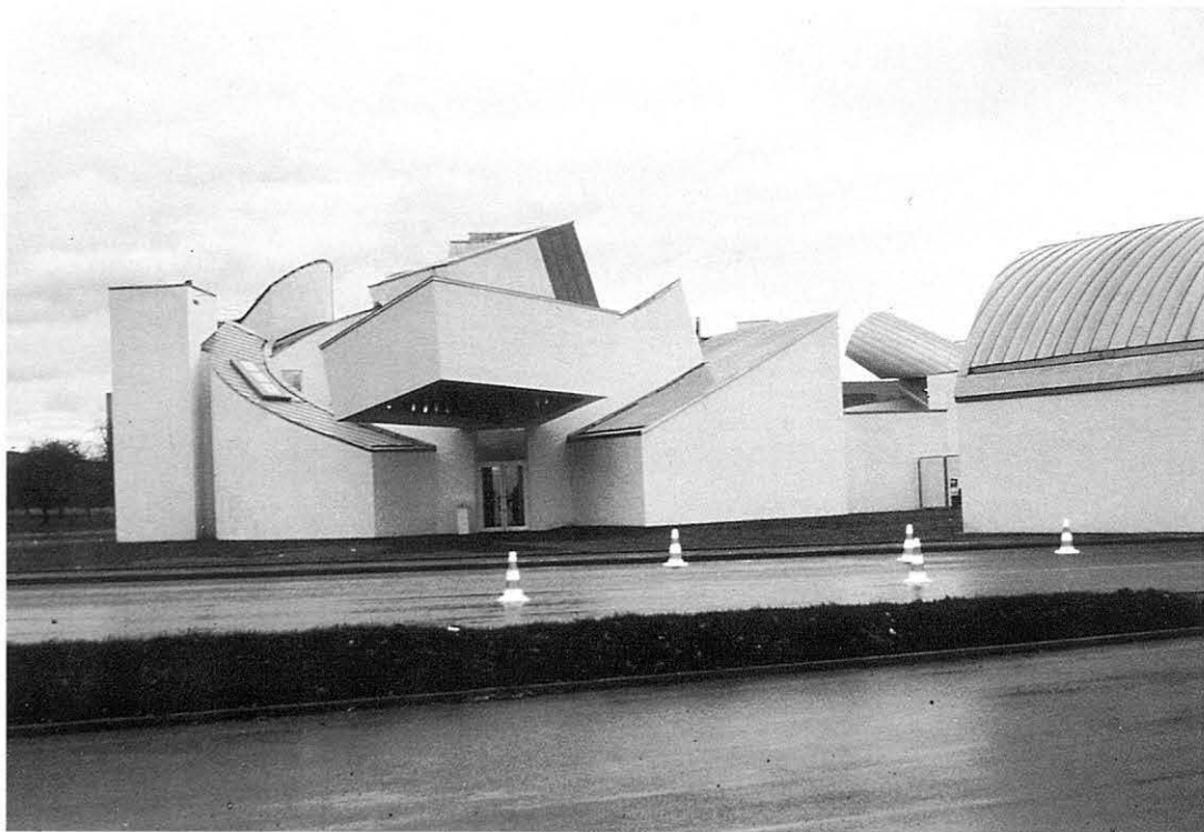
Exterior nord del Museu North view of the Museum
