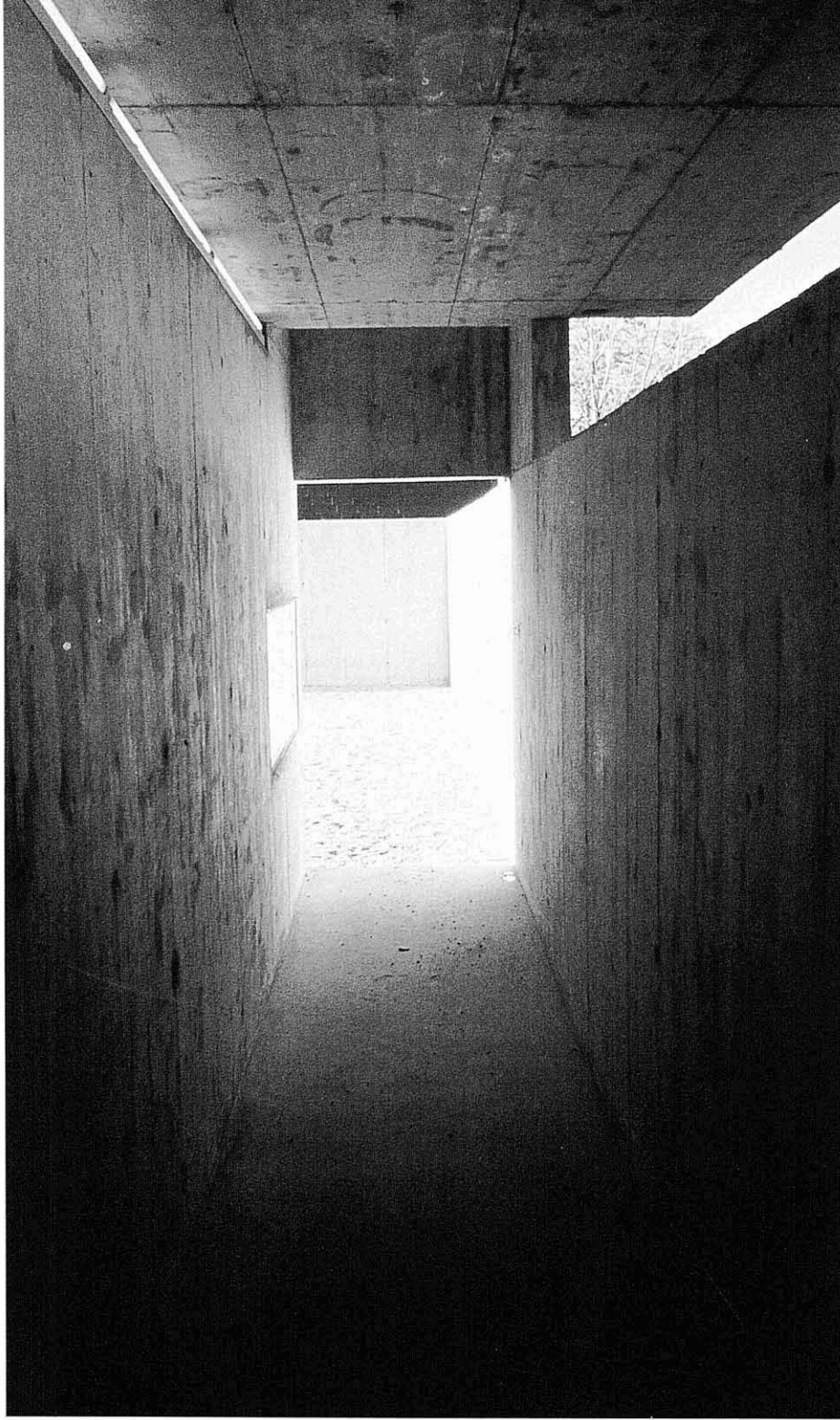
Pasillo entre la entrada principal y el patio. Corridor between the main entrance and the courtyard.
