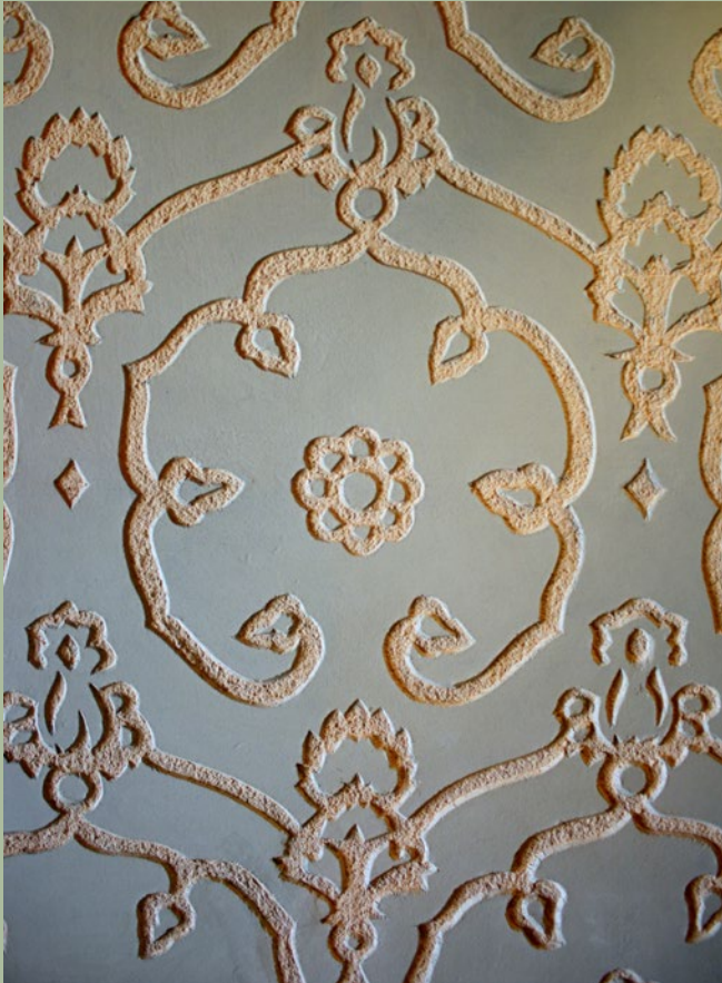
Detail of sgraffito in the entrance hall of Casa Garí (1899-1900), in Argentona. ©Daniel Pifarré.
