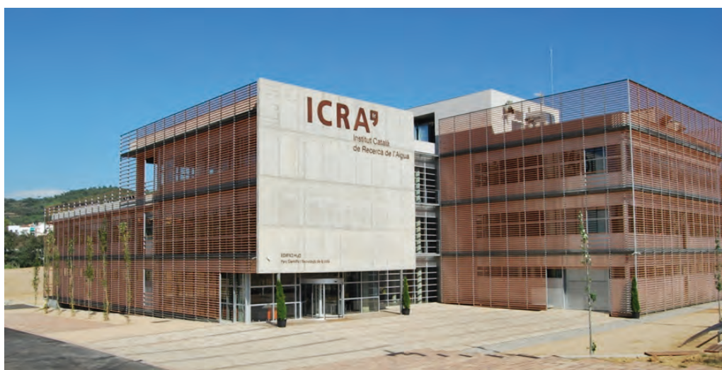
Fig. 1. The H 2 O building of the Catalan Institute for Water Research (ICRA), Girona.
