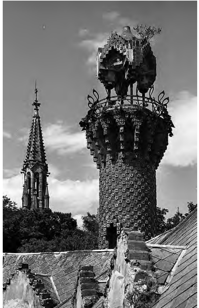
FIGURE 1. The tower of El Capricho and the belfry of the chapel of Sobrellano. Comillas (Cantabria). Photo: Antoni González (1971). GMN Archive.
