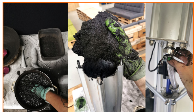
Figure 4. Mixing of ashtan and filling the tank of the 3D printer Source: Tin Wilke
