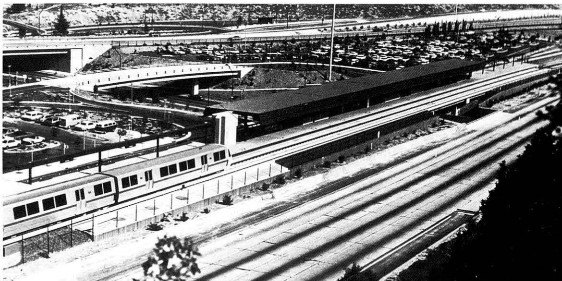
Lafayette Station of the Bay Area Rapid Transit, San Francisco (Architects: Gwathmey, Sellier and Crosby, J. Esherick and Ass.)
